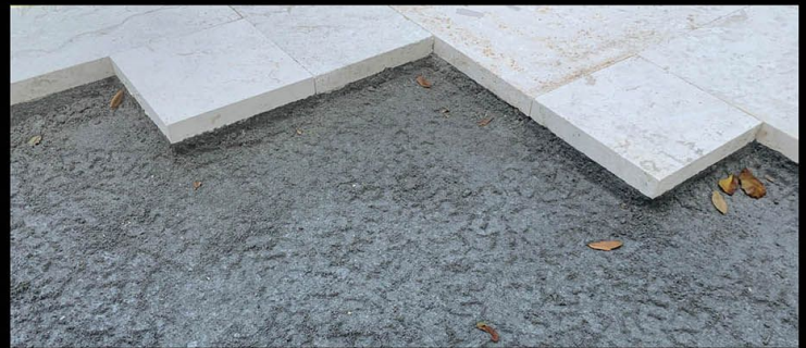
5- Mix Portland cement with sand and Anti Hydro and spread 2" thick.
