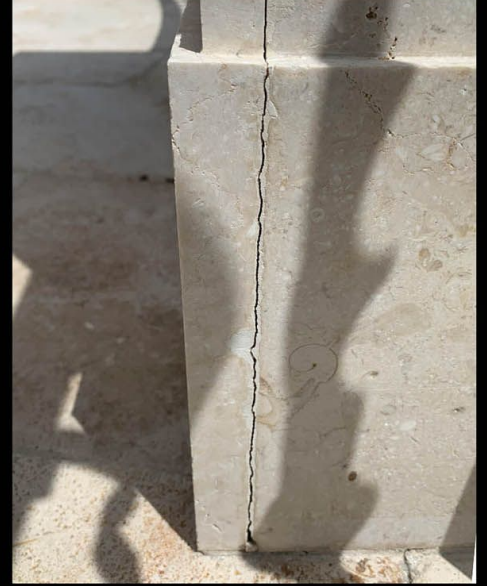
Epoxy cracking.
