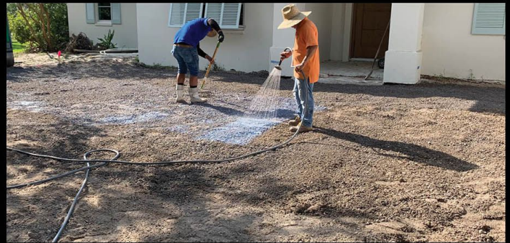
3- Spray Base Stabilizer and rake to go deeper.
