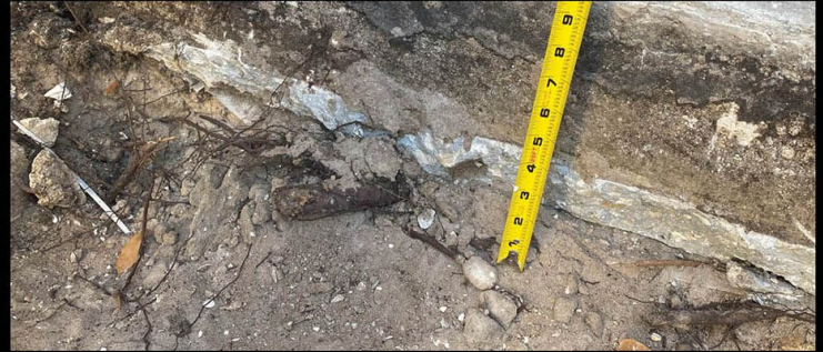
1- Remove 8" of dirt for pool deck installation (12" if driveway).
