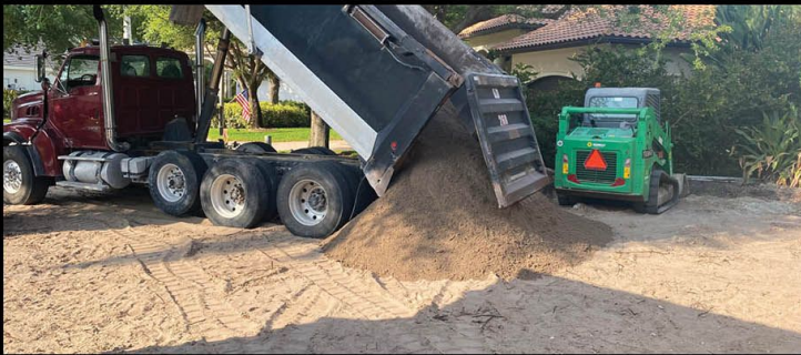
2- Dump and screed 4" of lime-rock for pool deck installation (8" if driveway).
