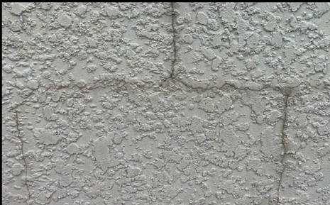
Stucco cracking.
